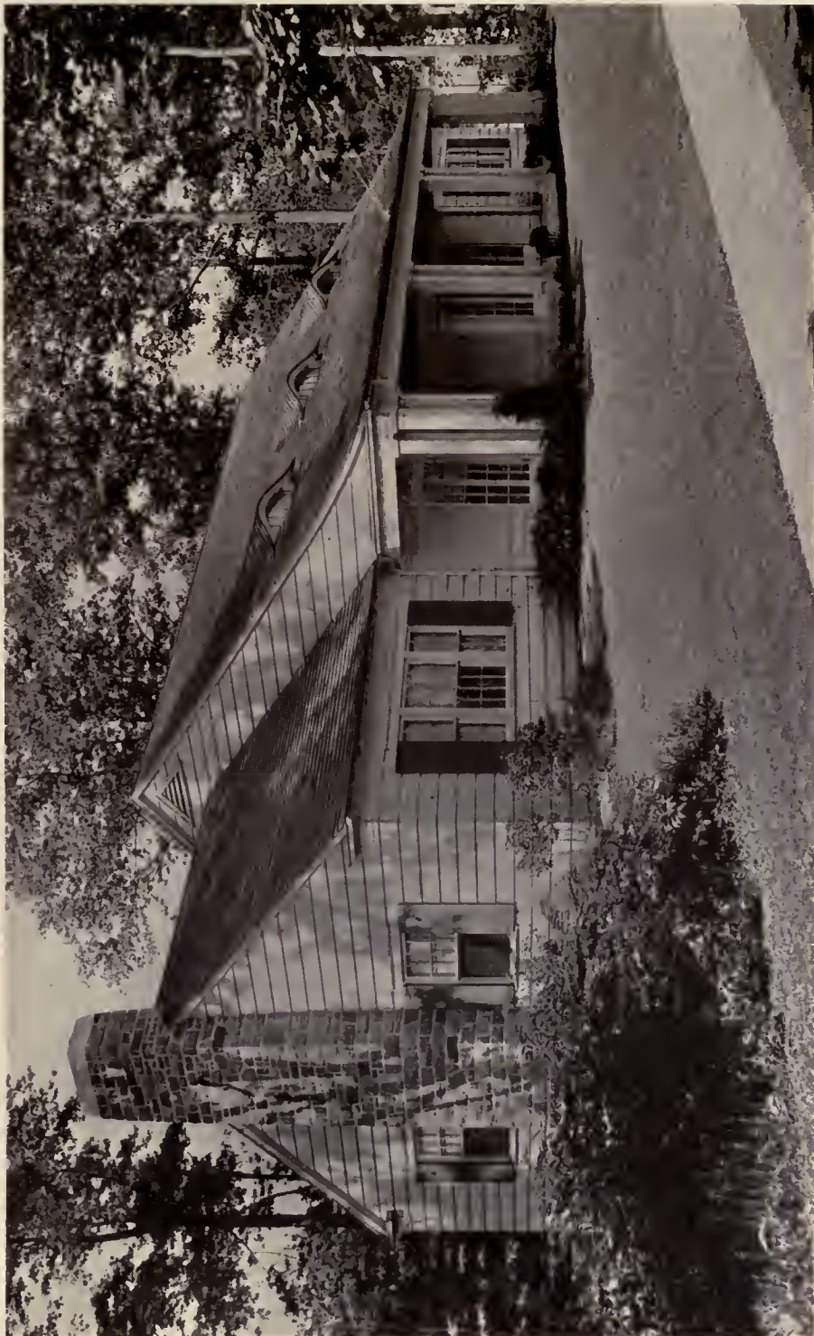
STREET VIEW RIVERDALE COUNTRY CLUB, RIVERDALE, N. Y. DWIGHT JAMES BAUM, ARCHITECT
